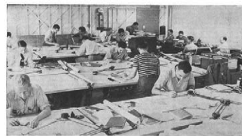
Time-saving monomorphism, which made possible design and construction of P-80 in just 142 days, was handled by MG mobile built and
