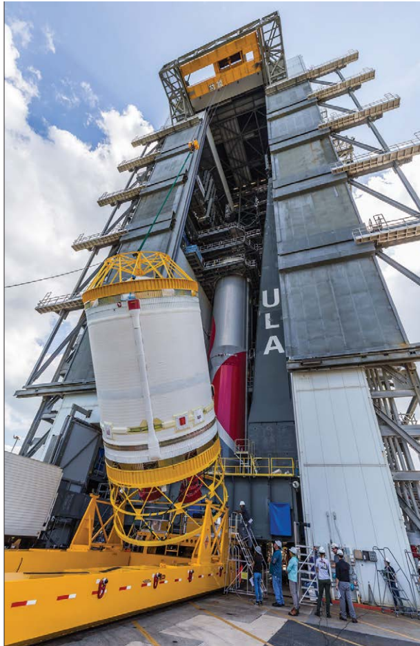
This Centaur V, pictured being hoisted atop the Vulcan Cert-1 booster in the Vertical Integration Facility at Cape Canaveral SFS Launch Complex-41 in February, was previously assigned to fly the first Vulcan mission. It will be retrofitted and reassigned.
