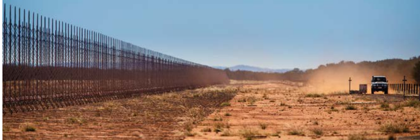
A receiving array of one of the three Jindalee radars in the Australian Outback.
