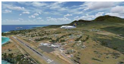
Nevis Island Amory International (TKPN) in the Caribbean's Lesser Antilles sports a single runway (10/28) just under 4,000 ft. long with a displaced threshold landing west end, as seen, high terrain to the south. Elevation of the runway is just 13 ft.
