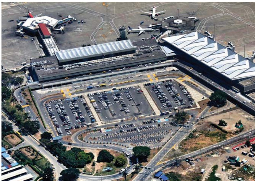
Cali Alfonso Bonilla Aragon International (SKCL) is located deep in a valley at 3,162 ft. elevation with mountain ridges rising to 15,000 ft. and 17,000 ft. on either side. Thus, maneuvering to sole Runway 1/19 is limited, as the valley constricts, and spatial orientation is crucial.
